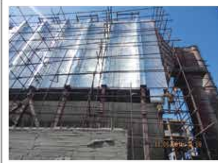
BMR Equipment in its Installation Phase
