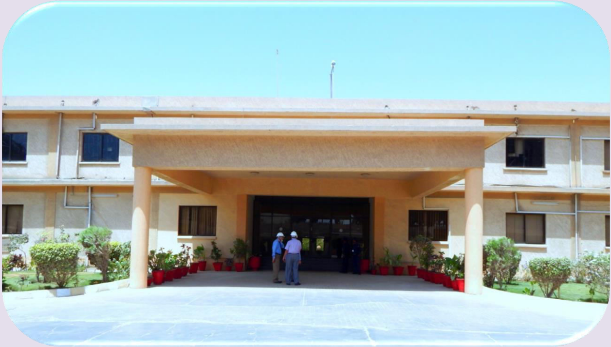
CCR Building of TCCL Plant (Venue of BOD Meeting)
