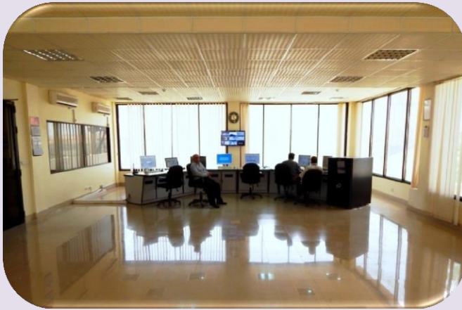
Central Control Room (CCR) - TCCL
